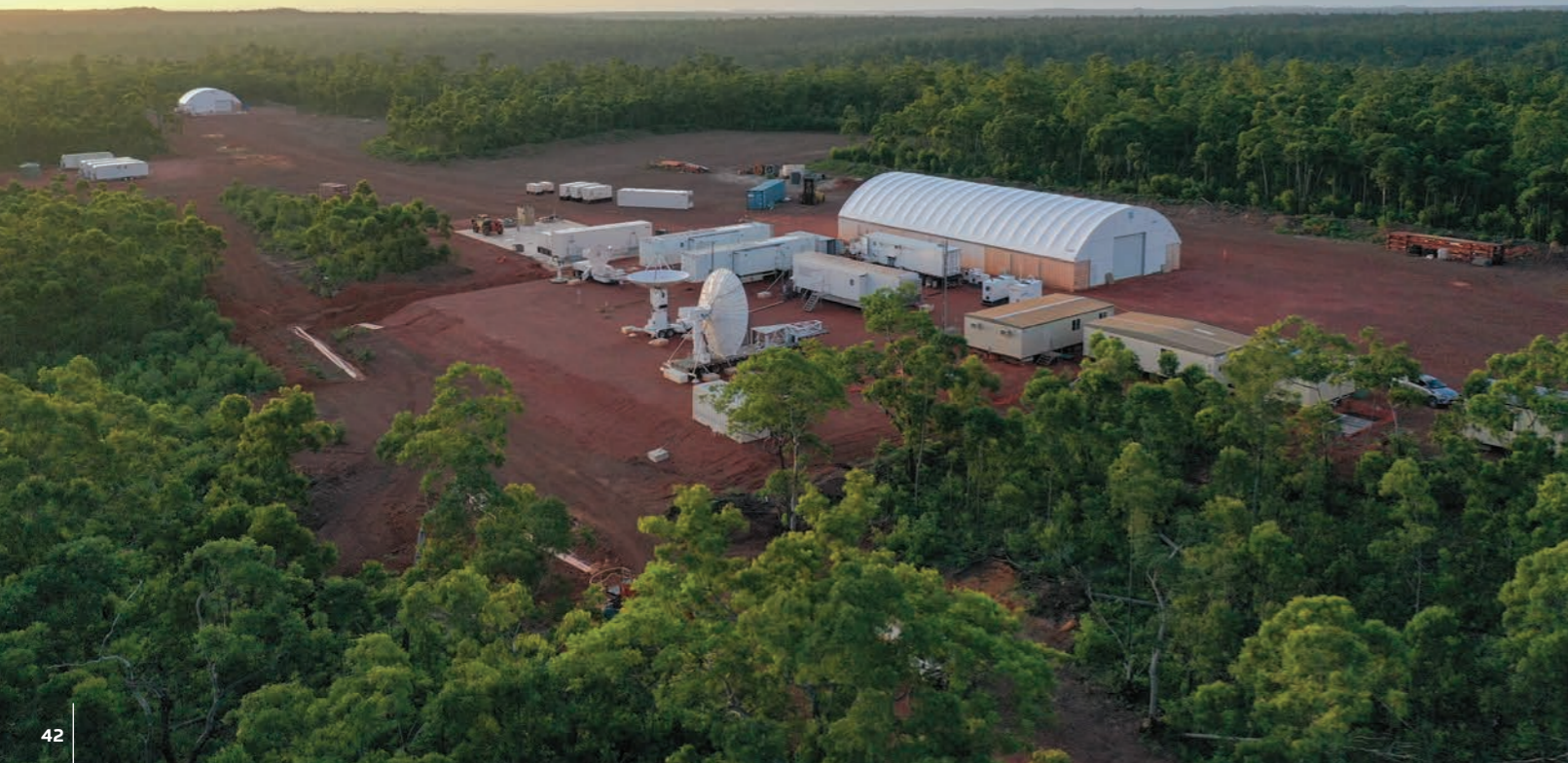
Arnhem Space Centre Horizontal Integration Facility
